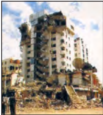
Fig. 3.3a: Destruction caused by an Earthquake in Gujarat
