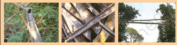
**Picture 2 and 3:** The channel sections, made of bamboo, divert water to the plant site where it is distributed into branches, again made and laid out with different forms of bamboo pipes. The flow of water into the pipes is controlled by manipulating the pipe positions.
